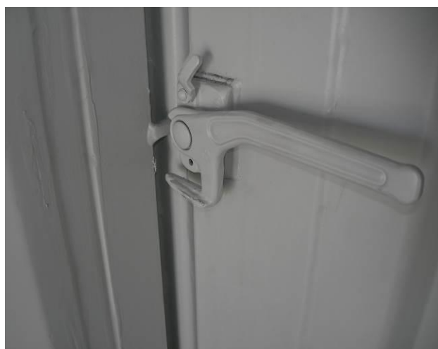
Fig 4. Bolting mechanism with handle for hinged door (from the inside)
